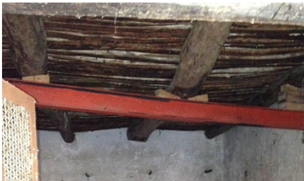
Figure 9: Ground floor slab with wooden trunks.
