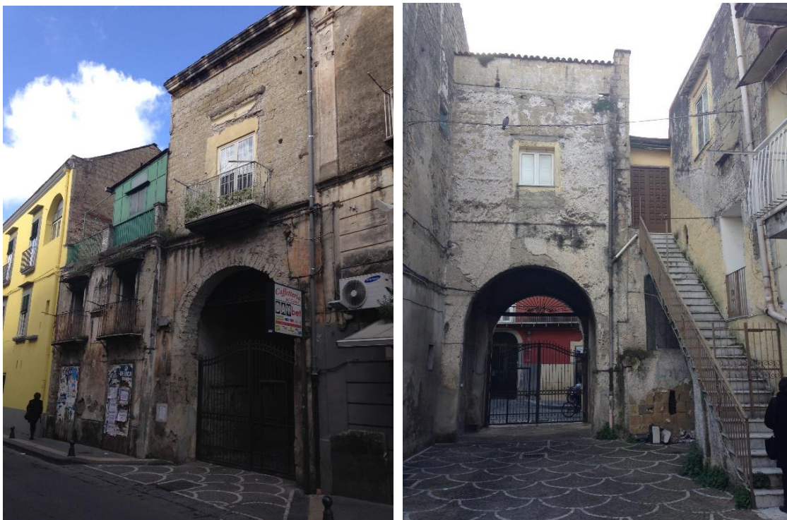
Figure 4: South view (left) and north view (right) of the case study.
